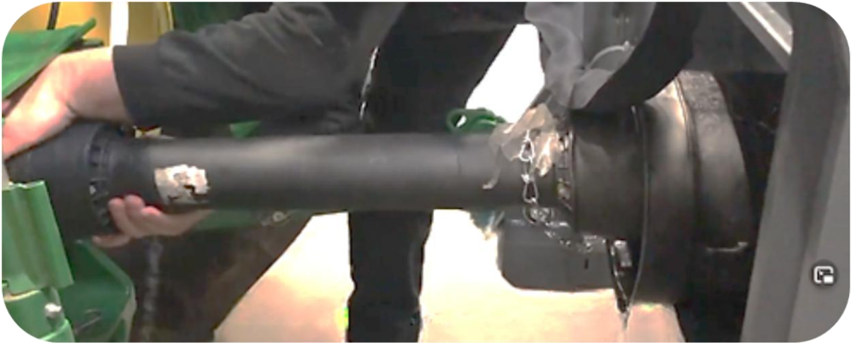
Installation of PTO shaft between Scorpion 490 boom mower and vehicle
